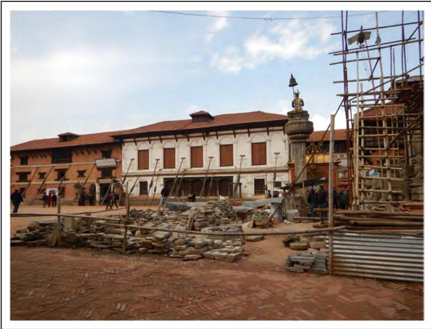
**Figure 6.** Overview of Durbar square and palace complex with the Malla-period palace (on the left) and Rana-period Lal Baithak shored up with wooden supports, January 2016. Photo: Katherine Hacker.
